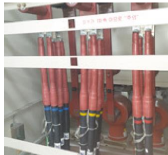
Hyundai Steel 154 KV Main VCB Panel, 33000V ACB Panel
