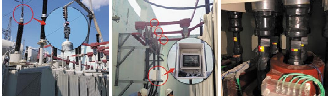
KEPCO Jinju Trasforming Station 154 KV T/R Bushing, Lead-in Busbar, Unmanned Transforming Station Power line
